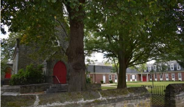
Historic Stone Church from Court Street
