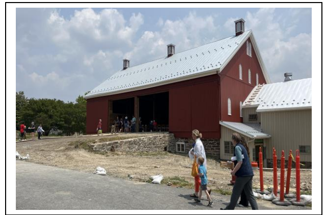
Renovation of the historic 1898 Barn for additional meeting spaces & dining
